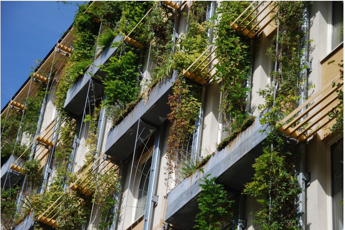
Figure 7: Example of plant-trough-based façade greening system with climbing trellis © Weiss-Tessbach
